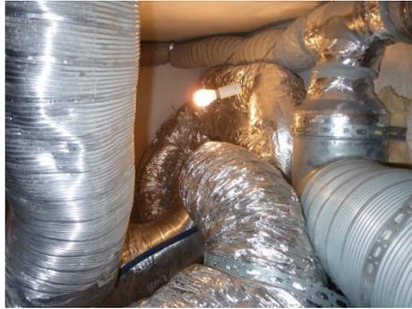
Figure 3: Example of observed defects in the ductwork of a high performance building ([www.programmepacte.fr](http://www.programmepacte.fr))
