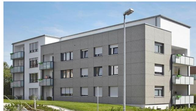
Figure 4: After retrofitting (KfW Efficiency House Standard 55), Pforzheim
